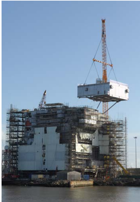
Living Quarters Helicopter Hangar installation on 23 rd October 2009
