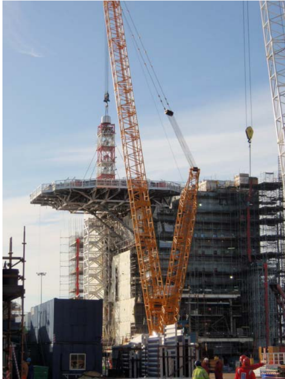
PH Living Quarters having the Helideck Lifted into position on 4 November 2009.
