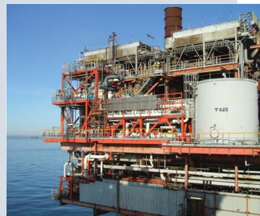
The completed Inde Project
